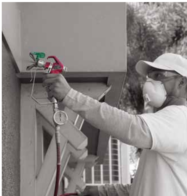
Latex emulsion paint through a standard 517 tip at 1,000 PSI
